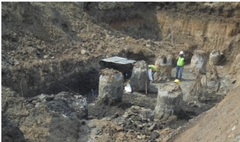
Figure 8. Soldier Pile Foundation
