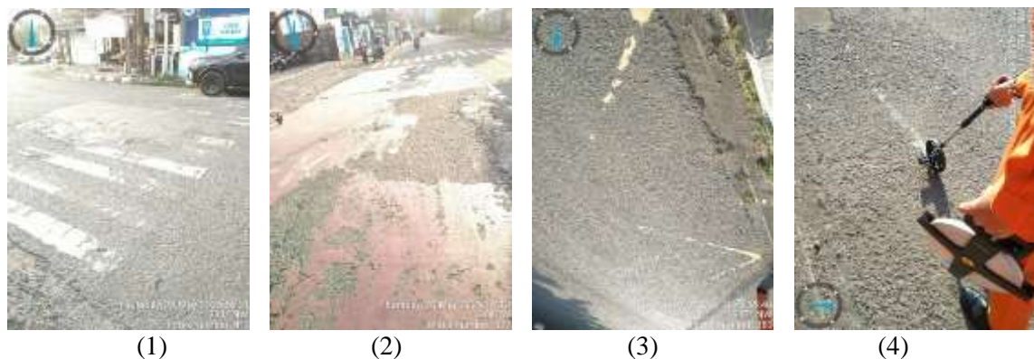
Figure 4. (1) Faded zebra crossing markings (2) ZOSS markings paint peeling off (3) Faded no-parking markings (4) Faded road shoulder markings
