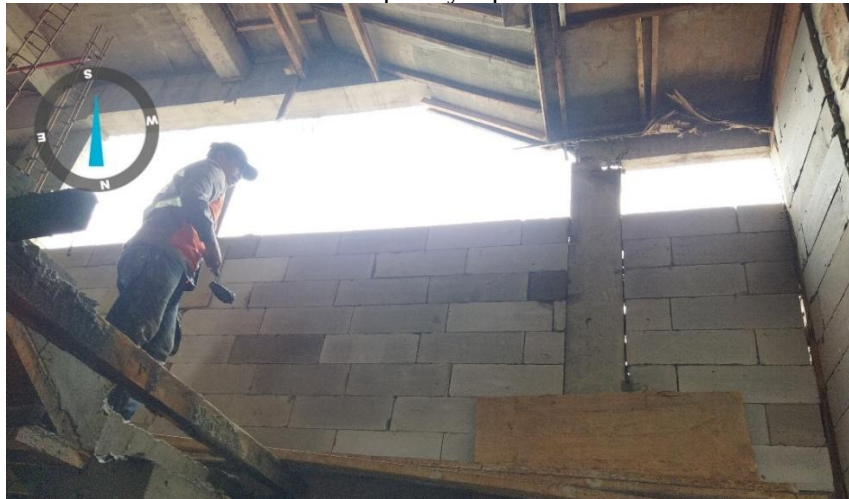
Figure 2. Lightweight Concrete Block Installation Work
