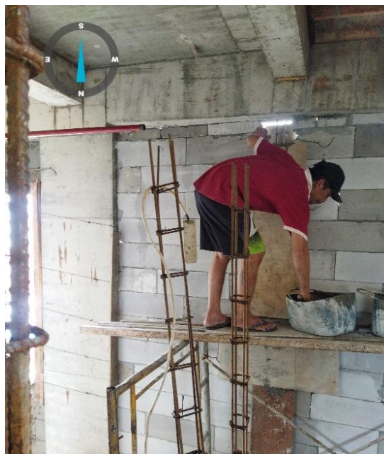
Figure 3. Lightweight Concrete Block Installation Process
