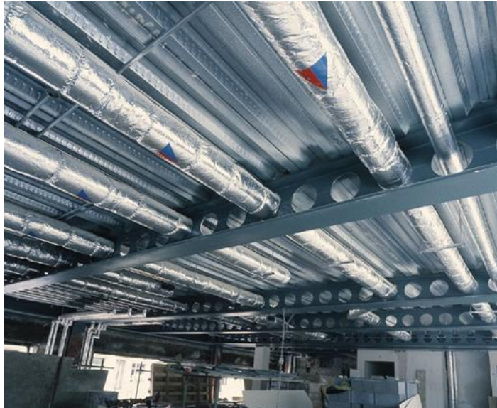
Figure 1. Application of Perforated Steel in high rise building (reff : http://www.steelconstruction.info )
