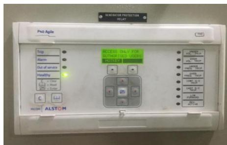
**Gambar 2. Relay Proteksi Generator Micom P342**
