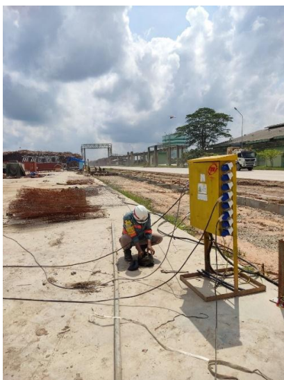
Gambar 19. Lokasi Pemasangan Panel SDP di Woodyard 2 Fabrikasi Material Power Boiler
