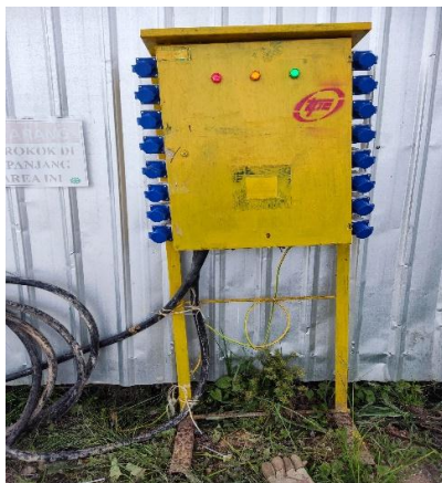
Gambar 18. Pemasangan Panel SDP di Woodyard 1 Fabrikasi Material Power Boiler
